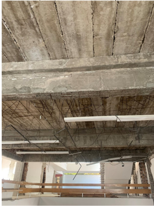
Figure 8. Beams and slab conditions of the NGA building
