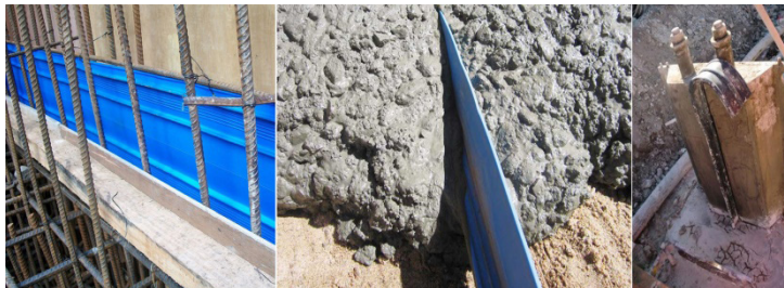
Figure 3 Flexible waterstop joint
