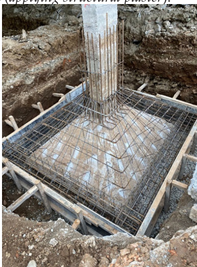
Figure 4. Excavated basement and foundation strengthening
