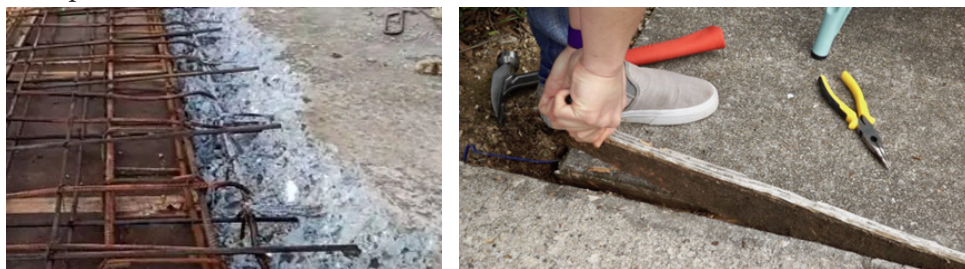
Figure 1 Realization of construction joints during pouring of concrete
