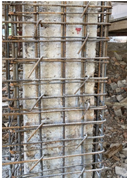
Figure 5. Columns were hammered and drilled to install the new rebars
