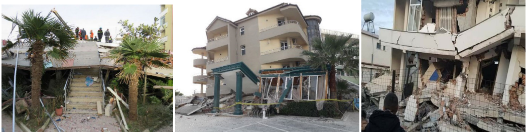
Figure 1: Total collapsed buildings
